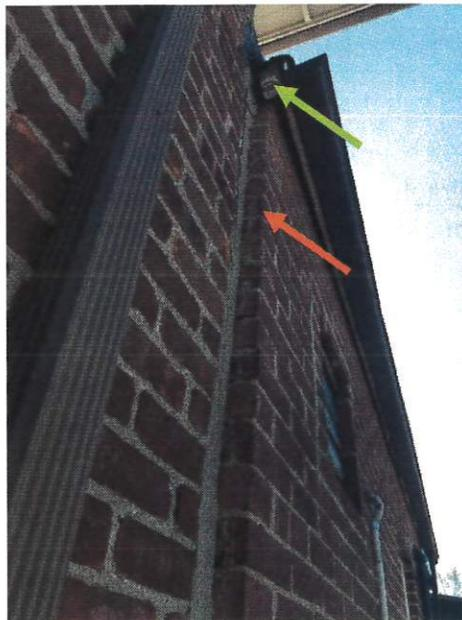
Photograph (7): Reported displacement at kitchen addition (red arrow). Deteriorated wood curb / blocking (green arrow).
