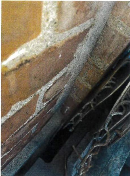
Photograph (8): Kitchen addition masonry aligned with lower concrete parge coat of main building. No evidence of significant displacement (leaning) after construction.
