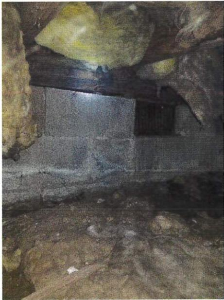
Photograph (19): Poorly supported sill plate. Displaced insulation. Representative conditions.
