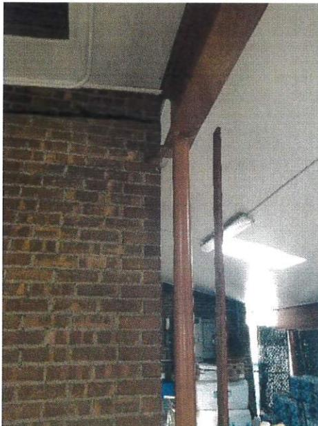
Photograph (9): Damaged brick masonry at canopy steel.
