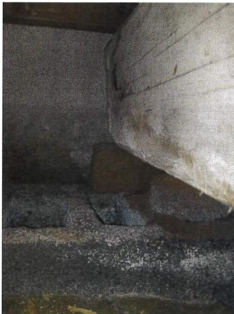
Photograph (17): Poorly supported earring condition at center girder (north end).
