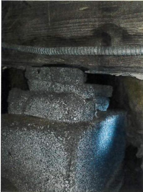
Photograph (16): Poorly supported bearing condition at center girder (mid-span).
